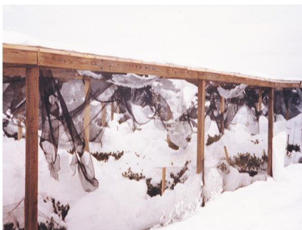
Figure 15. Disasters: (left) snowstorm with cut shade cloth, and (right) twisted house structure from the snow storm of January 2000.
