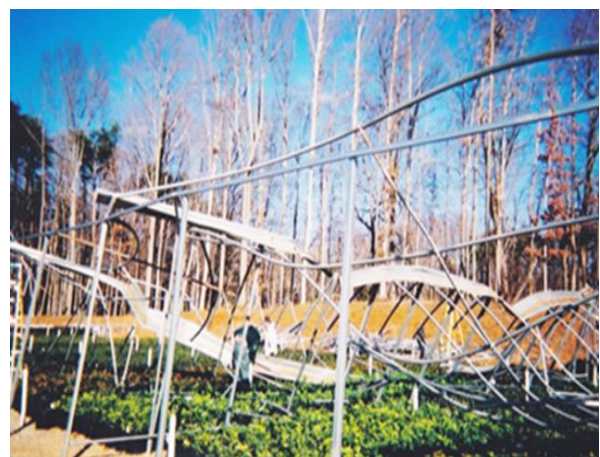
Figure 15. Disasters: (left) snowstorm with cut shade cloth, and (right) twisted house structure from the snow storm of January 2000.
