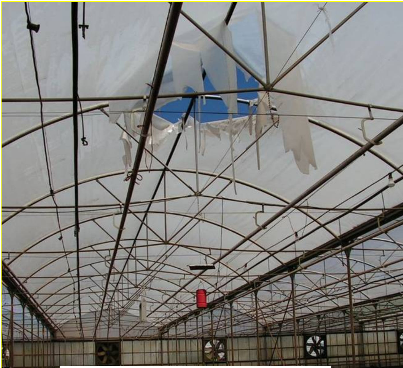
Film degradation- sulphur evaporation
