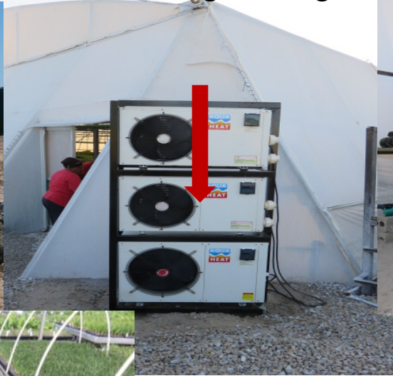
Heat pump heating water during the night
