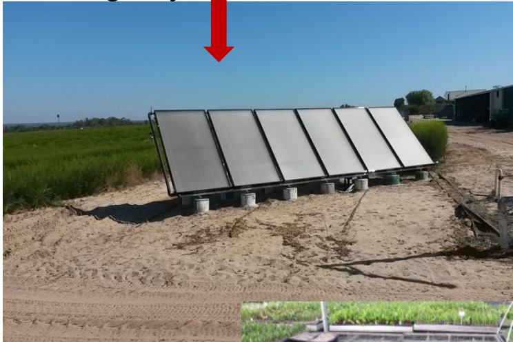
Solar panels heating water during day
