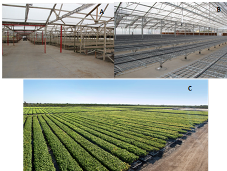
Figure 7. (A) Old type greenhouse with wooden benches over dirt floor; (B) Modernized greenhouse; and (C) modernized outdoor growing area, both constructed with steel benches and concrete floors to minimize pathogen exposure to the plants.
